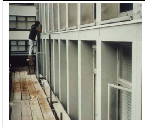
Figure 1b Cosmetic overcoat applied
